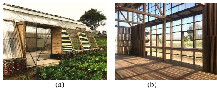
Gambar 5. a) Bangunan Training Hall; b) Ruang Restoran (Sumber: Archdaily.com , Diunduh: 21/06/21 – 11:38)
