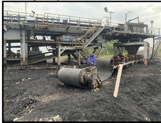
Gambar 3. Pengantian sabuk ban Belt Conveyor
