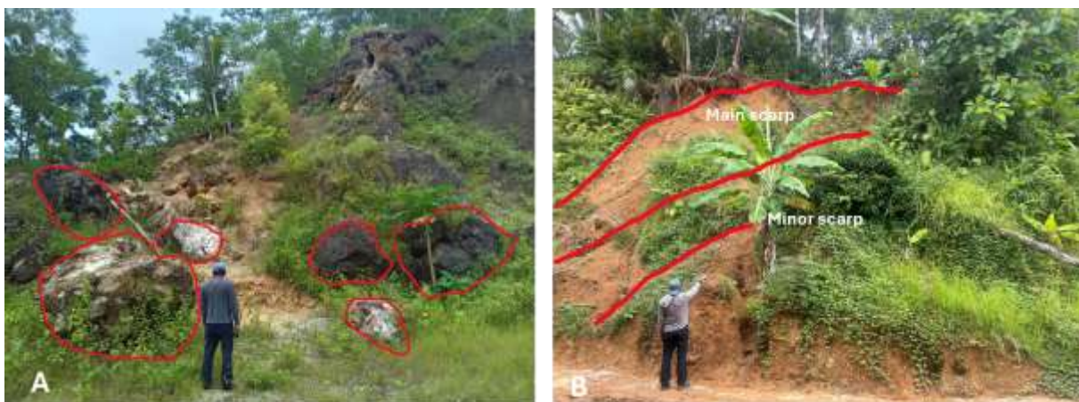
Figure 2. Landslide occurred in the study area (a) Rockfall; (b) Rock sliding
