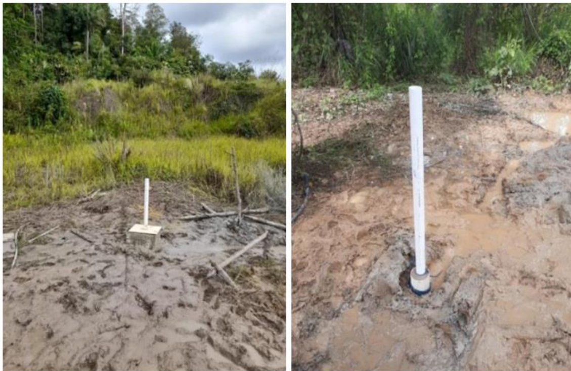
Figure 4. Groundwater drilling 1 (left), groundwater drilling 2 (right)
