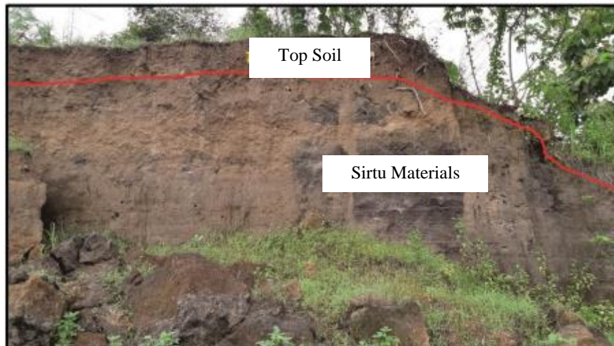
Figure 3. The appearance of the topsoil that covers the gravel-sand excavation material
