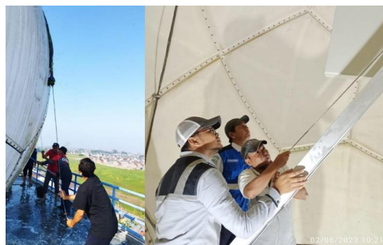
Fig. 2 Weather Radar Maintenance
