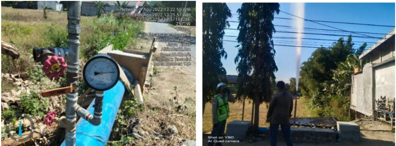
Fig. 5 Hydrotest implementation at the work site
