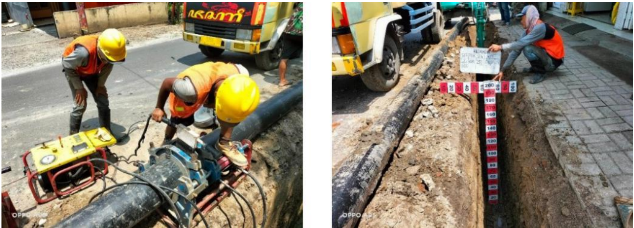
Fig. 3 Depth of HDPE Pipe Excavation and HDPE Pipe Connection
