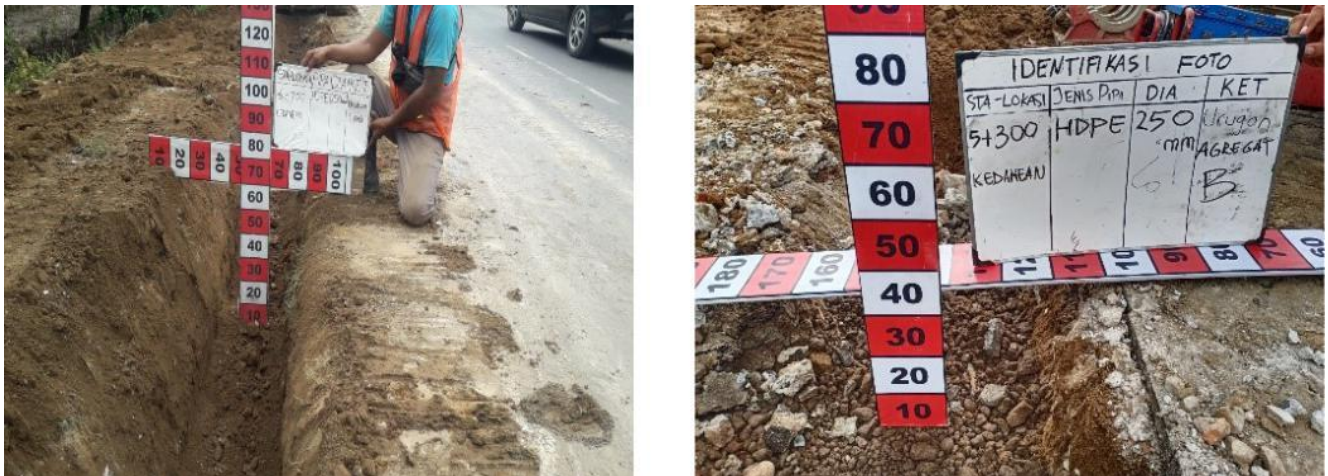
Fig. 4 Depth of HDPE Pipe Excavation and HDPE Pipe Connection
