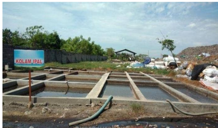
Figure 3. Leachate Reservoir Reactor
